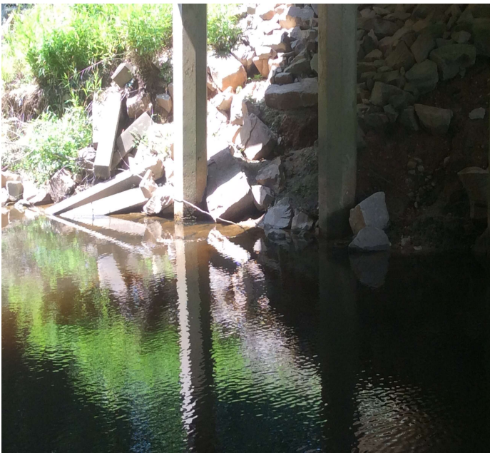
PHOTO 1 Description PILE 6 IS CRACK AT GROUND LINE 1/4 CRACK BENT 2 RIGHT SIDE
