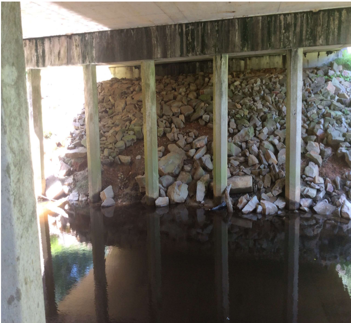
PHOTO 1 Description PAST FLOODS HAVE MOVED SOME OF RIPRAP FROM SLOPE UNDER SPAN 1
