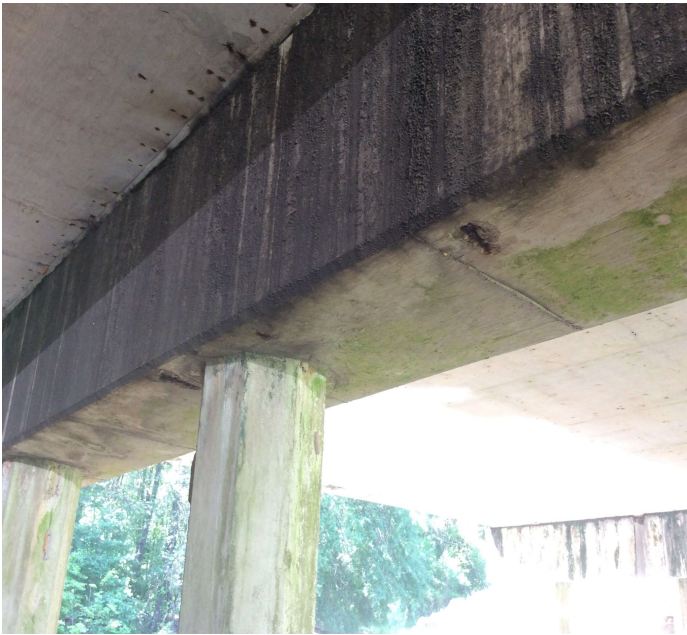
PHOTO 1 Description BENT 2 & 3 small SPALLS WITH REBAR EXPOSED
