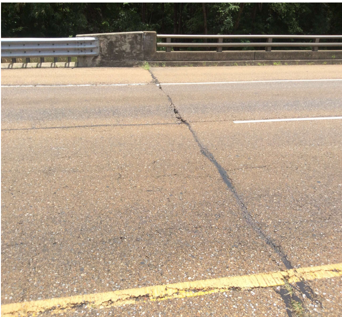
PHOTO 1 Description ASPHALT AT ALL JOINTS UNRAVELING AND FORMING POT HOLES
